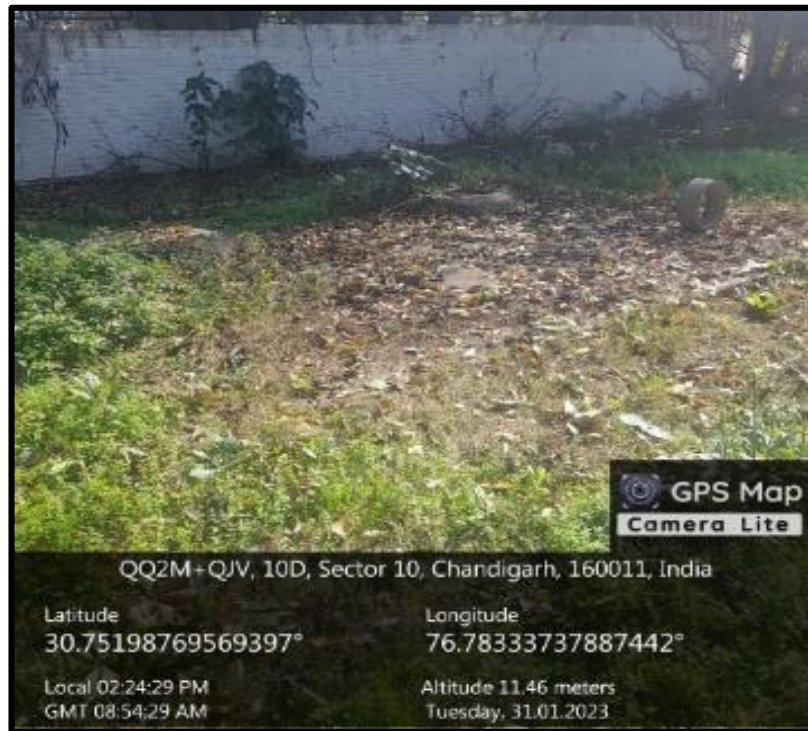
Collection pits having connecting from Rooftop to ground water through R.C.C. Pipes
