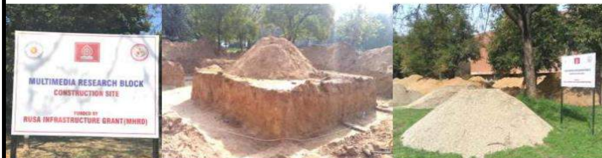
Multimedia Research Block— Construction Funded by RUSA (MHRD)
