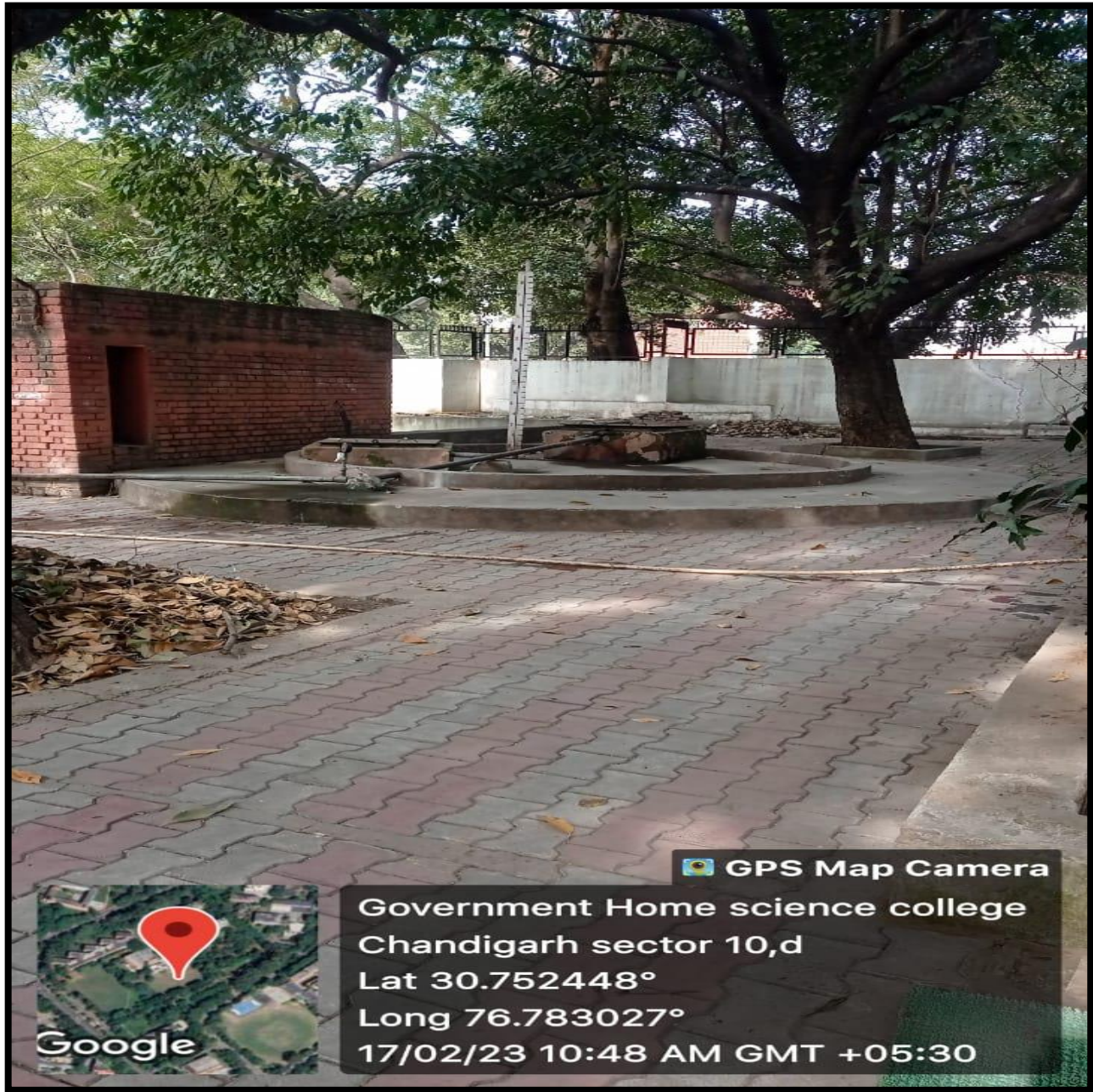
Water Boosting Station
