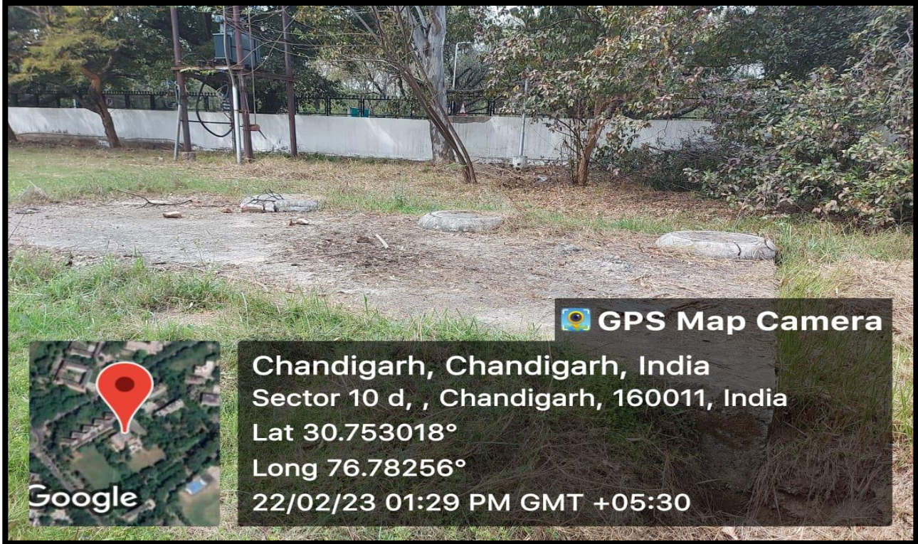
Rain Water Collection Pits
