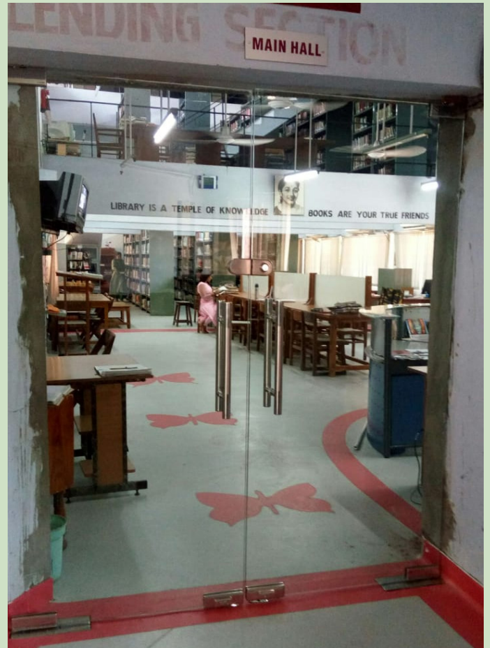
Library has been renovated with PVC flooring to reduce noise and glass doors to make cooling more effective so that conditions are conducive for learning and reading for students.
