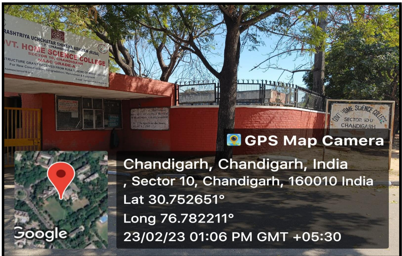
Fencing at Boundary Walls of The College
