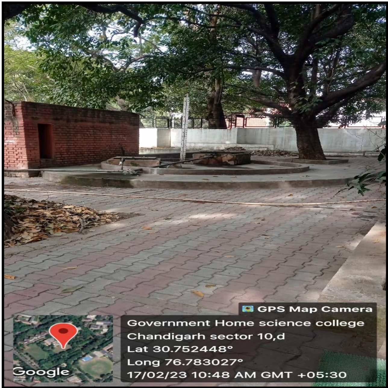
Water Boosting Station
