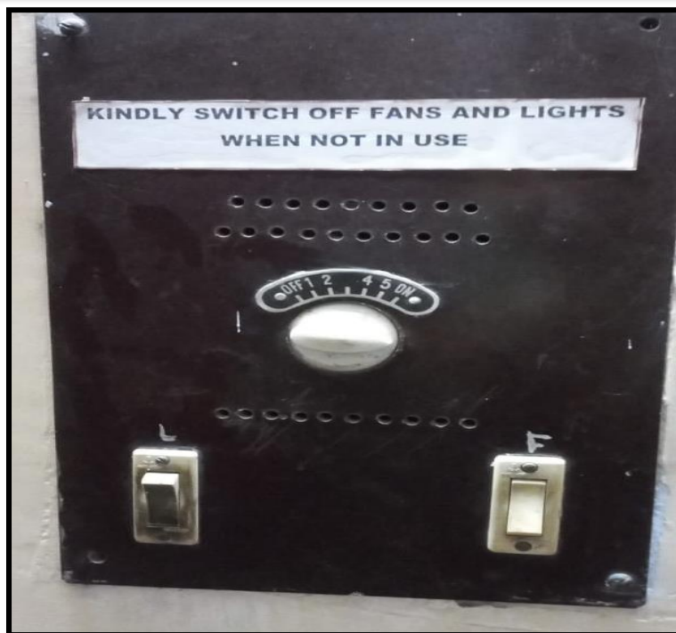
Display of Methods for Energy Conservation by Energy Brigade
