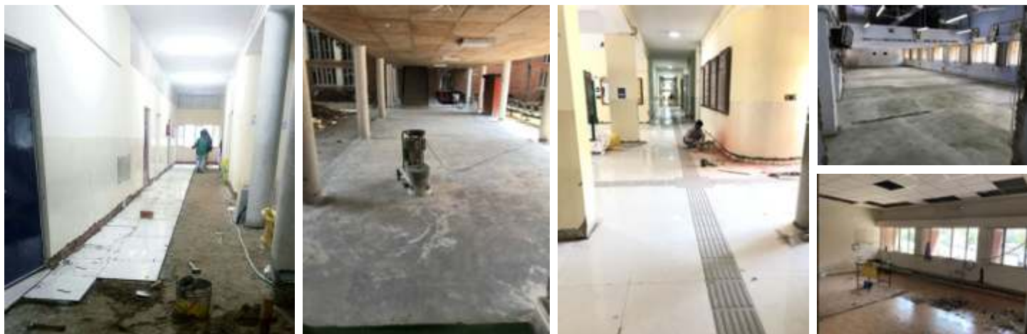
Disabled friendly tactile flooring of corridors
